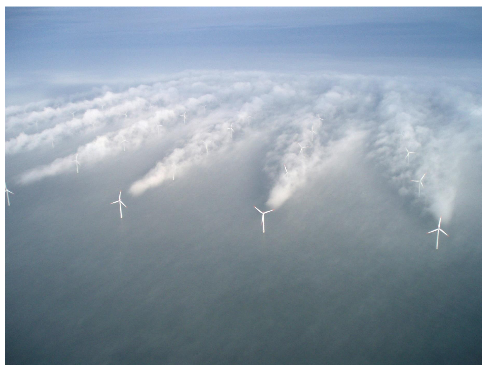
Vattenfall's Horns Rev 1 offshore wind farm. Photograph by Christian Steiness (https://millicentmedia.com/2012/09/11/cutting-costs-for-offshore-wind-farms/)
