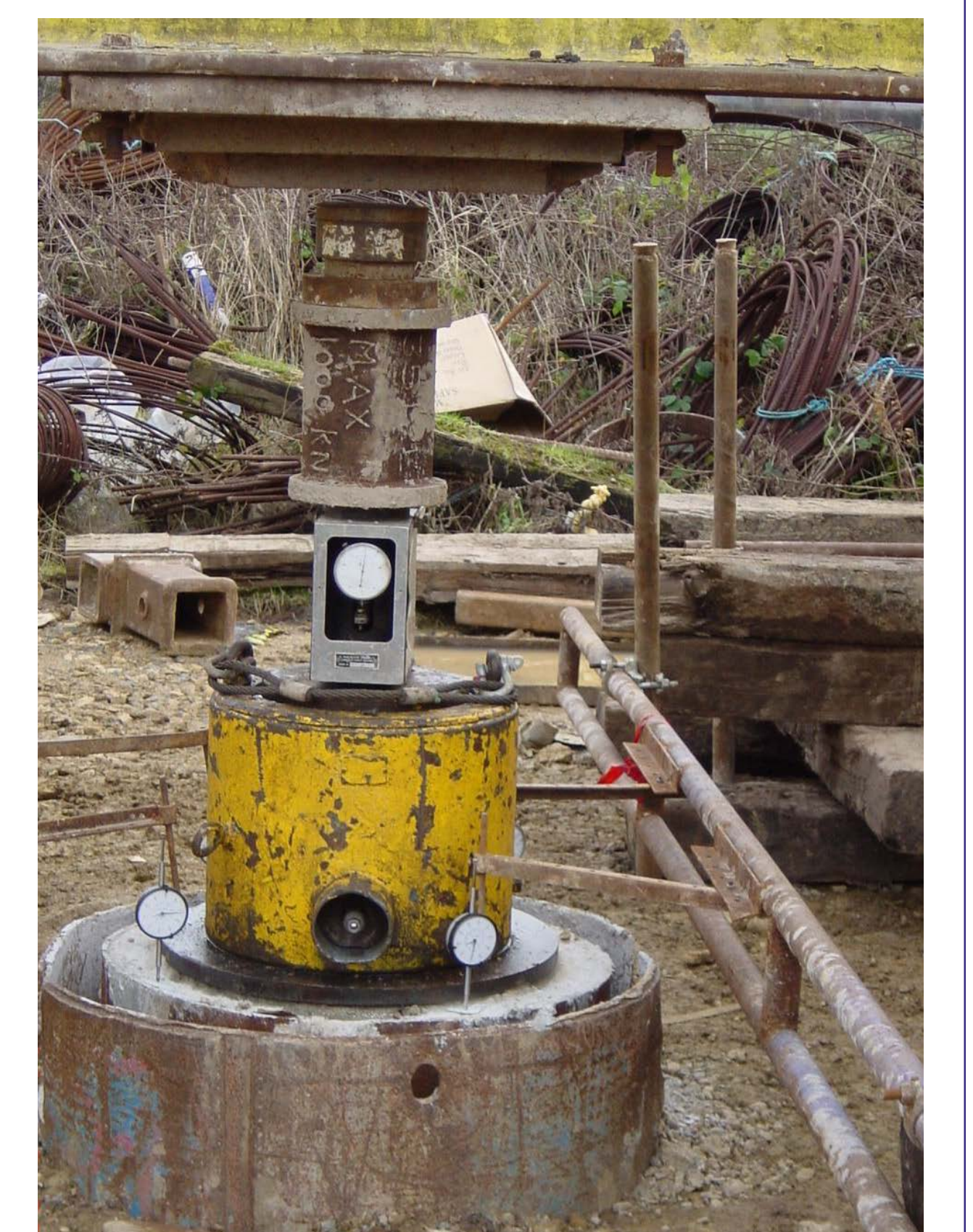
Figure 9. Example of field testing of pile capacity.
