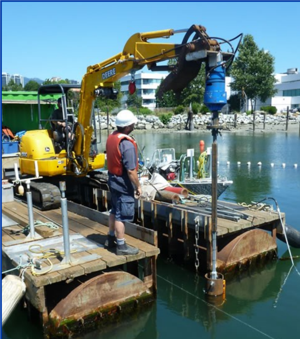
Fig.1: Screw pile installation for offshore
