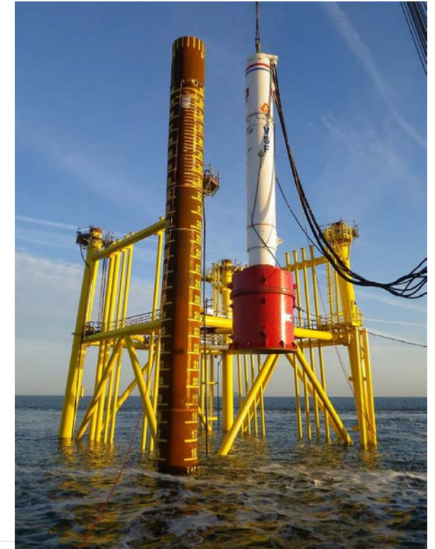
Offshore jacket installation (driven piling)
