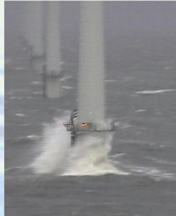
Wave run-up on one of the towers of the Horns Rev wind farm
