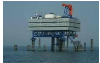
Horn Rev Offshore Substation
