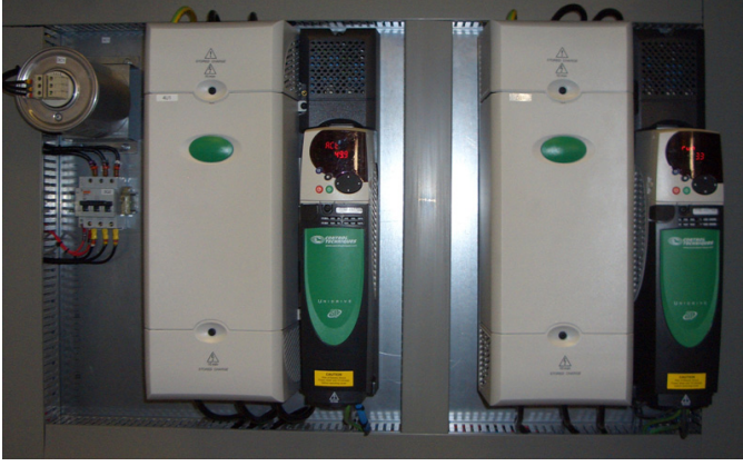
Fig. 2. Rotor circuit back-to-back converter
