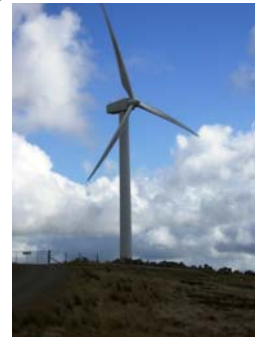
Fig. 1. 660kW Vestas V47 wind turbine, Hare Hill, Scotland
