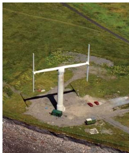
Figure 9. The Carmarthen Bay vertical axis wind turbine VAWT 850 (500kW) from the late 1970's.
